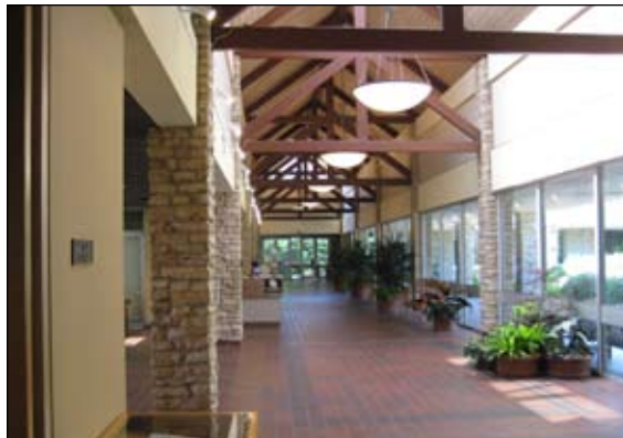
Existing entry area at the Garden Center - Provide improved information about the entire Garden
