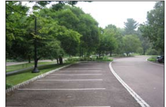
Morris Arboretum - Example of using a pervious surface to manage runoff in a parking lot.
