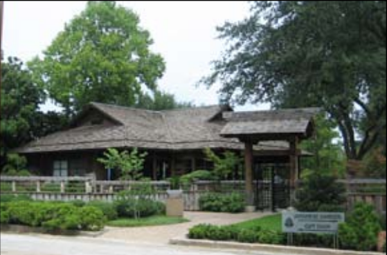
When the new gift shop is completed, the current gift shop in the Japanese Garden can be easily converted to an event space that will increase revenue to the Garden. This building has a beautiful setting with fantastic views of the Japanese Garden to the north.
